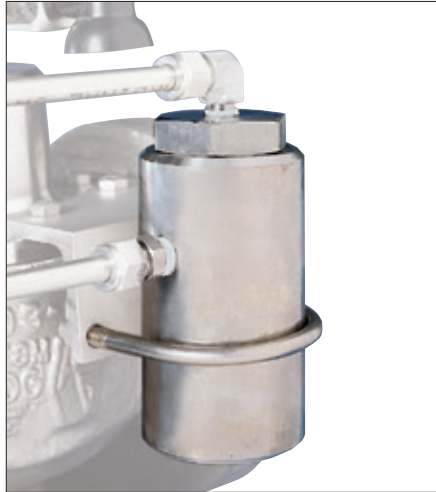
C. PILOT SUPPLY FILTER
